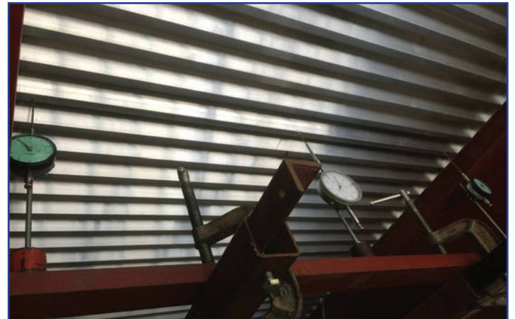
Internal View of Horizontal line load test
